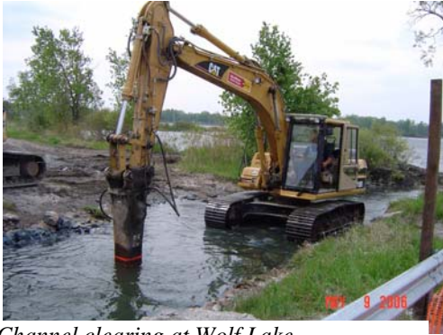
Channel clearing at Wolf Lake
